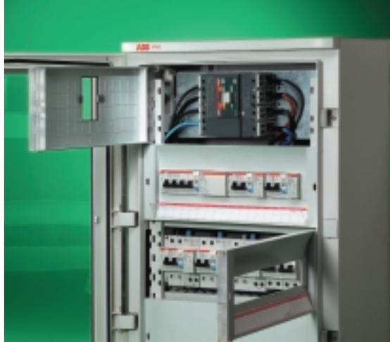
a hinge-on inner door. Further accessories such as the partial plates fitted onto the modular frame and the kit for installing molded-case circuit-breakers means that the switchboard can also be used for mixed distribution/automation applications.
