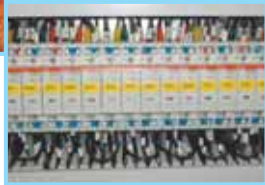
ESB20...ESB63 for control of lamp rows
